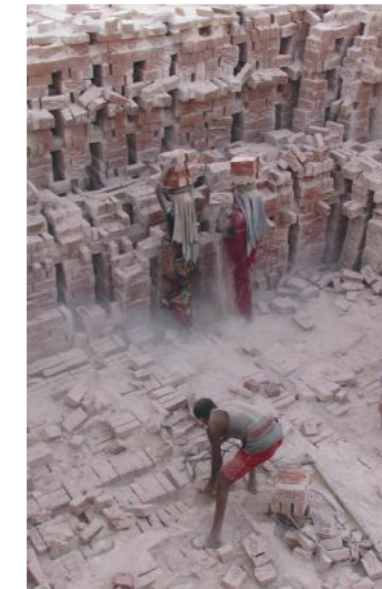
Unloading of fired bricks
